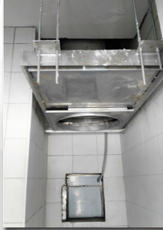
Cutoff door in the end of the chute
